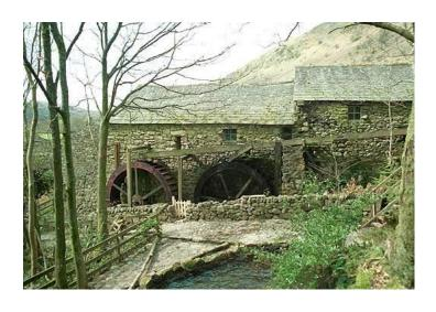
shoe, agitated by a 'damsel'. The meal or flour was used for animal feed or fed through an eccentrically rotating sieve for kitchen quality oatmeal. Oats where the main source of food for the valley down the centuries, although in more recent times the second wheel was added, with French stones for grinding corn. Many other pieces of machinery are on show at the mill and it is a fascinating insight into a bygone age.
